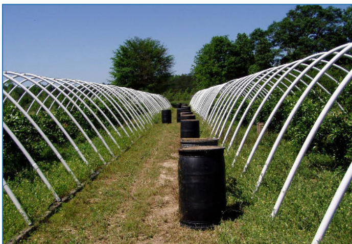
Figure 10. Arched hoops made of PVC pipe used to make a semi-permanent frame.
